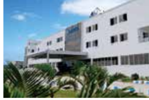
Rudrapur Plant (Green Building)
